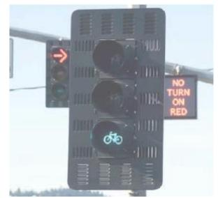
Figure 10: Bicycle specific signal head
